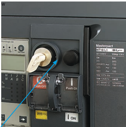
Electrical closing pushbutton BPFE.
